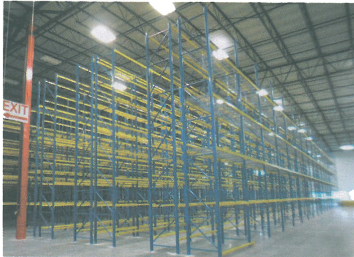
Meridian Design Build completed a 226,102-square-foot build out for Molto Properties and LASCO Fittings, Inc. in Romeoville, Illinois.
