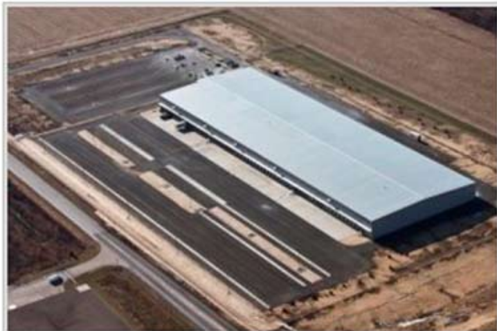
Rock Island Distribution Center
