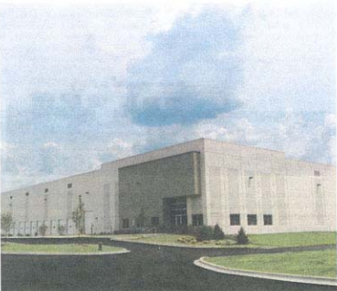
Meridian Design Build worked closely with developer DP Partners to incorporate sustainable design into their latest 495,000-sq-ft speculative industrial facility within LoganCenter at Sauk Village. Green design concepts include native landscaping, clerestory windows, T-5 fluorescent lighting, low VOC paints, and construction material recycling.
